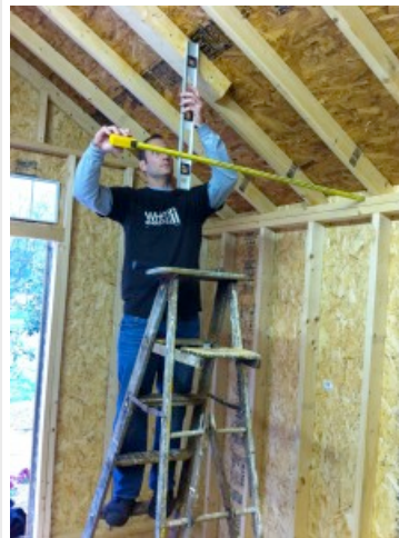
Workers build a storage space for Angels and Sparrows Soup Kitchen in Huntersville last month as part of the "What if Everyone," charity event. It was one of many projects volunteers took on across the region.
